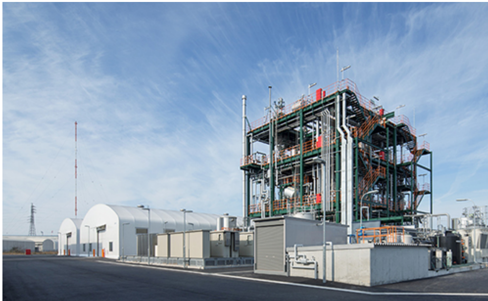
KHP (Kitakyushu Hibikinada Plant), a 2 kTA demonstration plant
